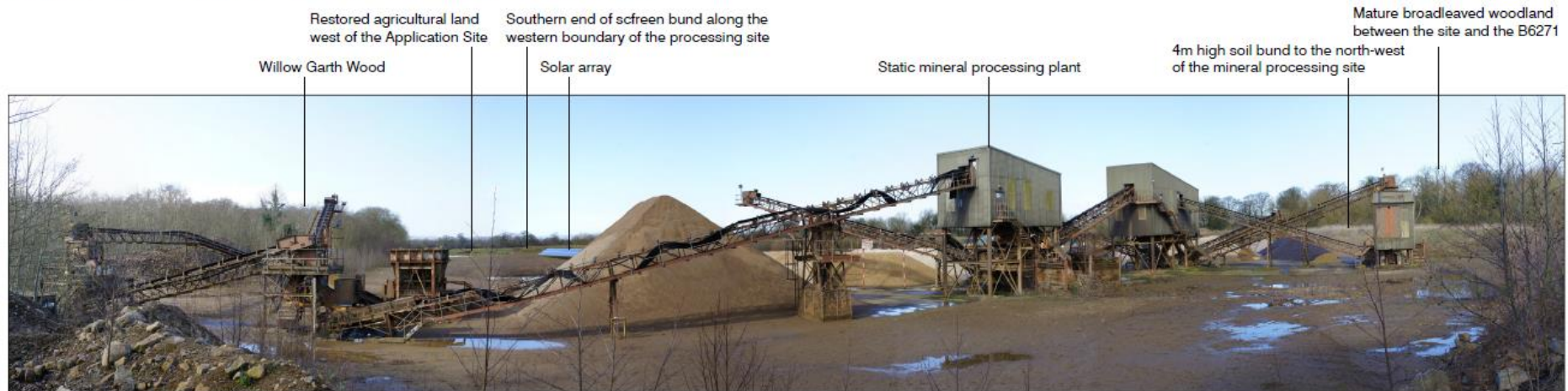
Viewpoint B: Elevated view to the west from the bund along the eastern side of the existing plant site
